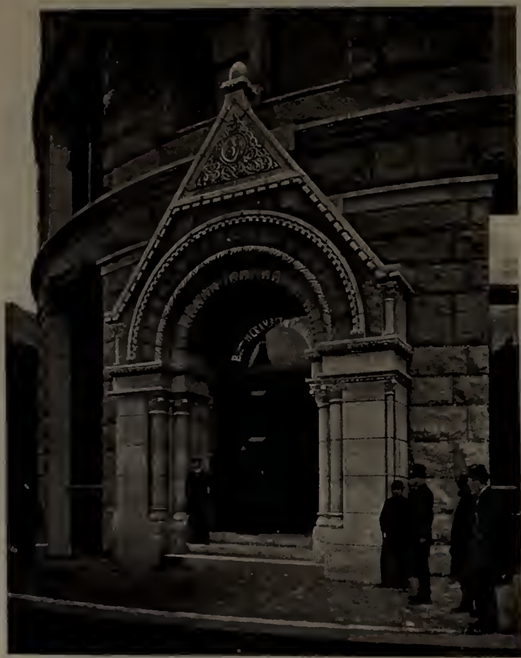
ENTRANCE TO THE CHAMBER OF COMMERCE.
